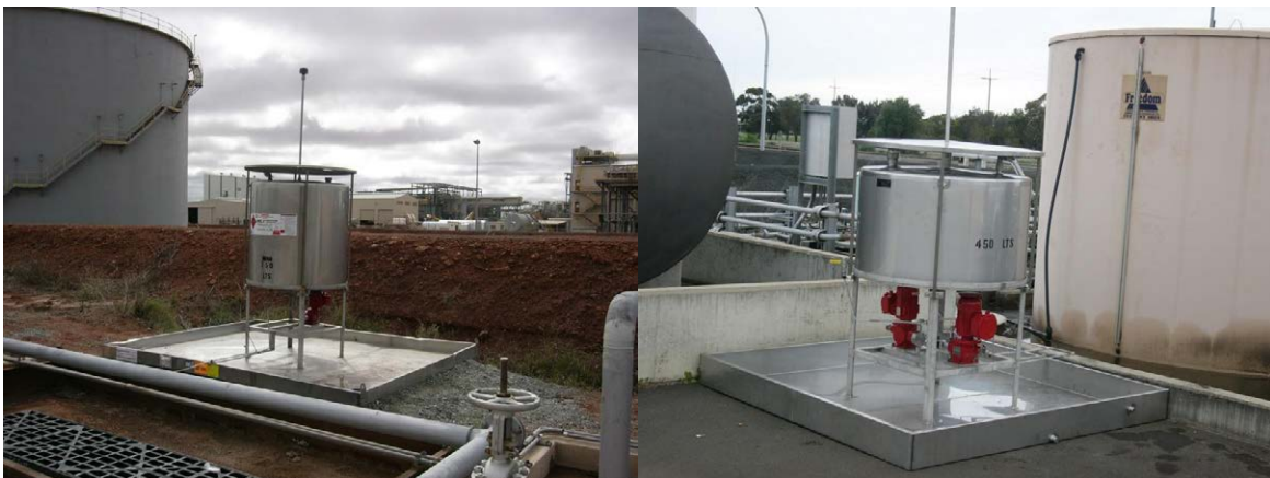
Automated dosing systems
