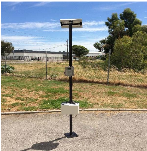
Remote solar powered dosing system
